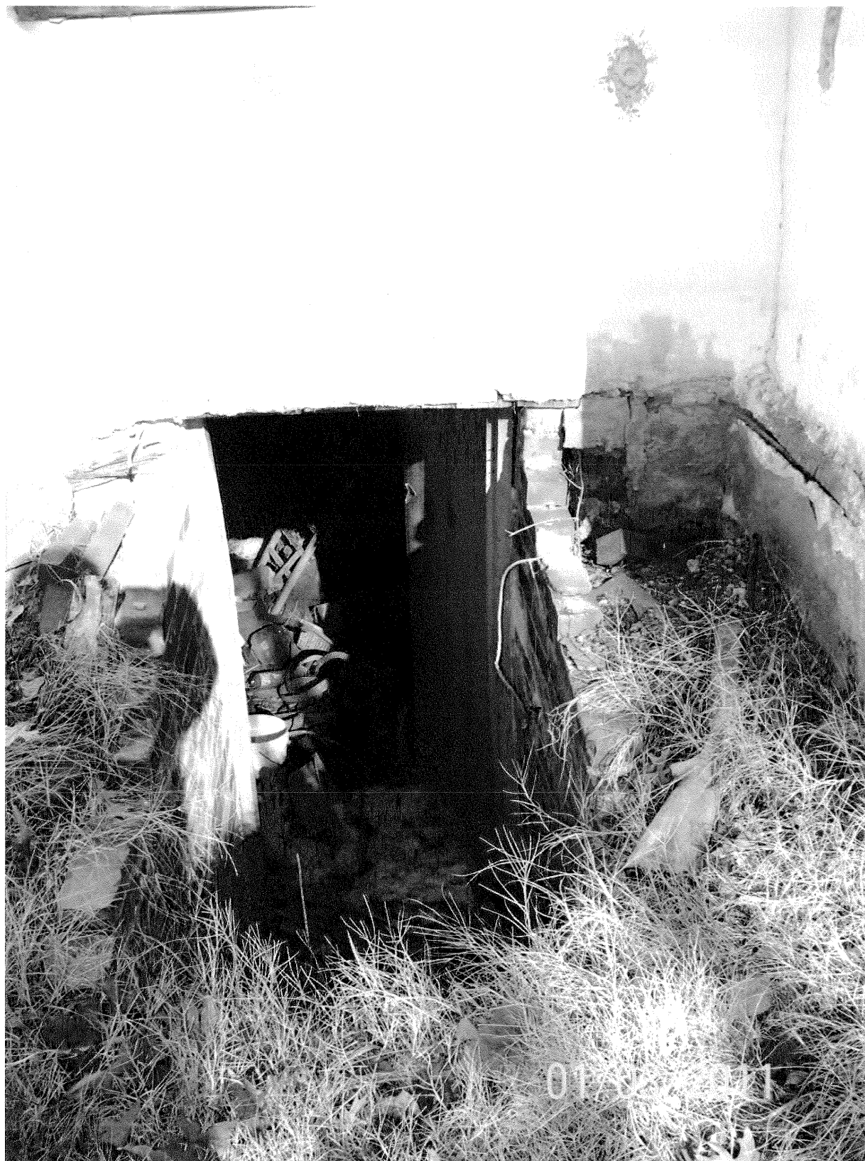
Basement of structure is open
