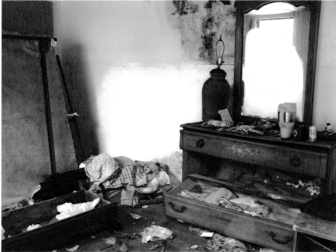
Accessory structure open, signs of previous occupancy
