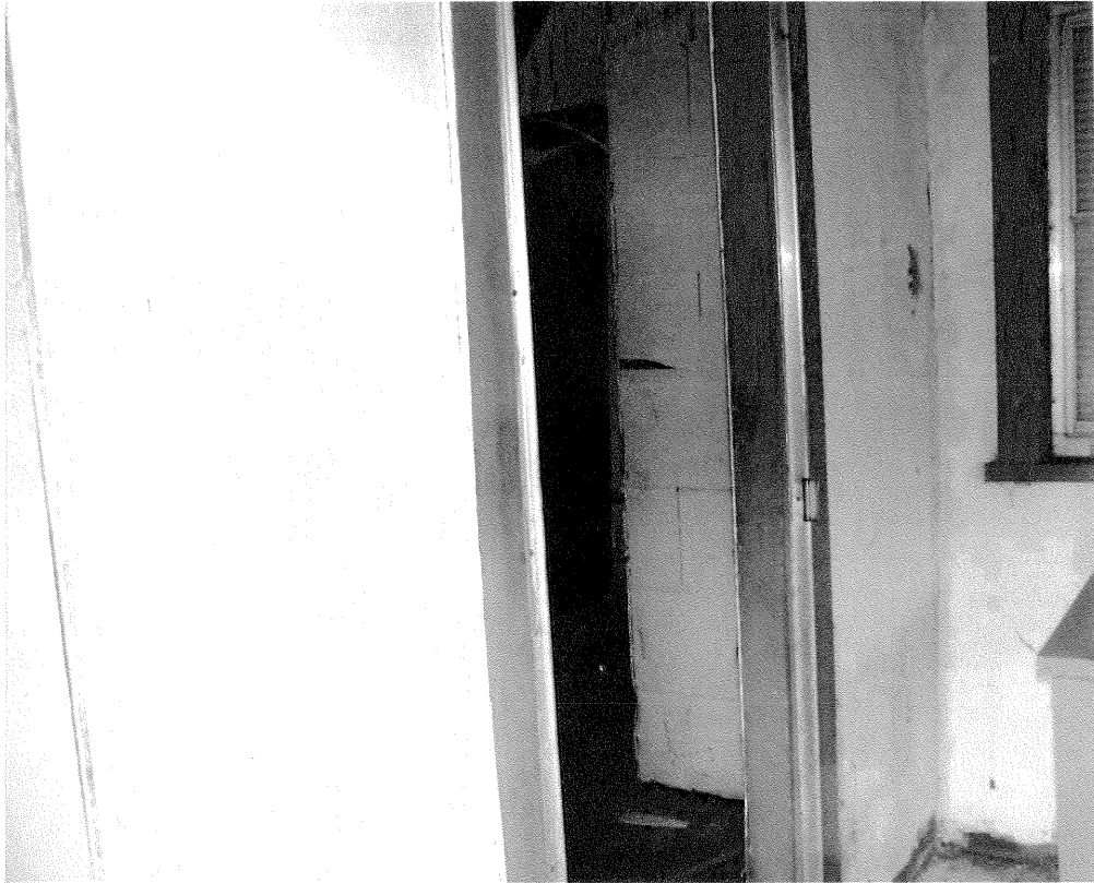
Rear window and door of structure open
