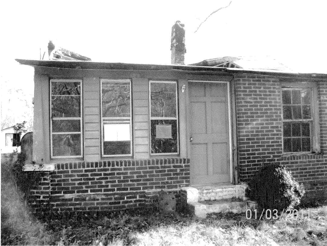
Front of single-family structure
