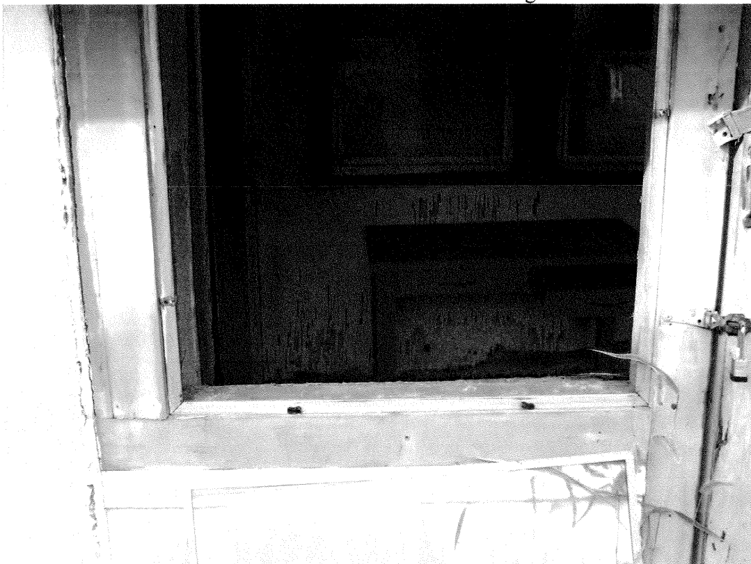
Rear window and door of structure open
