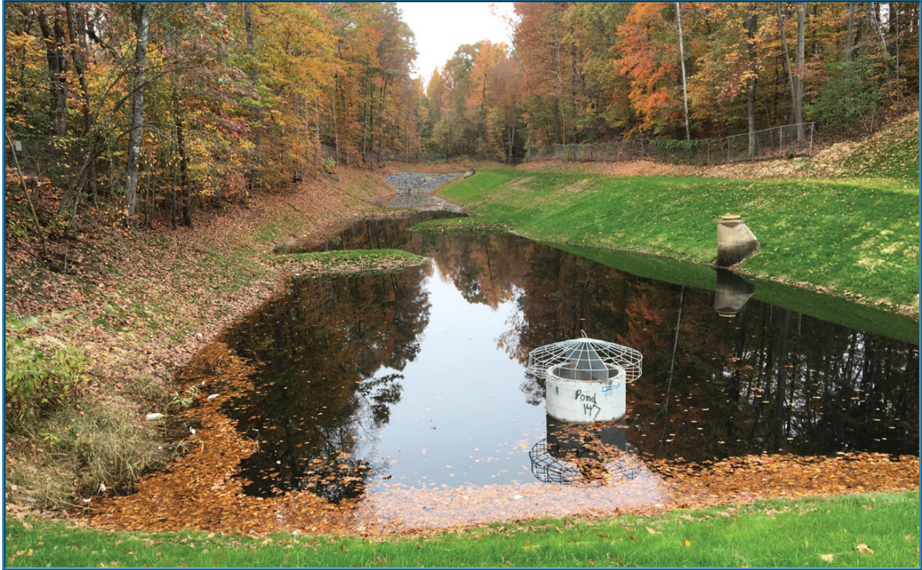
Powells Creek Watershed Water Quality Retrofit
