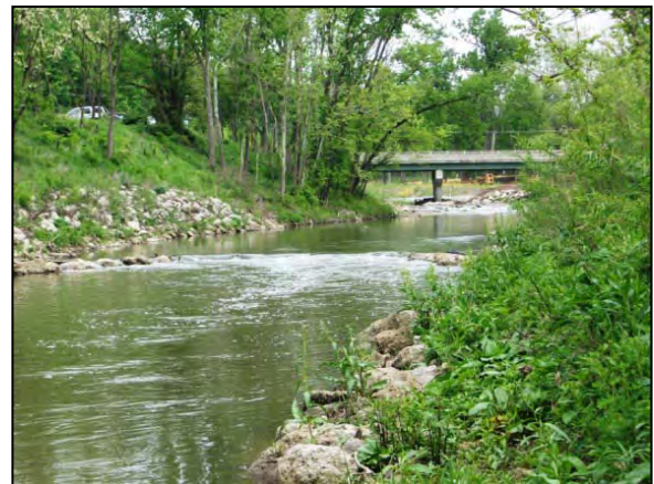
Figure 5-5: Rock toe bank treatment and in-stream structures downstream of bridge.
