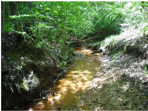
Figure 4-23: Deposition and channel widening, from Myrtlewood to Medford Drive, Reach 665-G.
