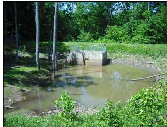
Figure 4-42: Wet pond lacking forebay, with adjacent forest cover, FAC-533.
