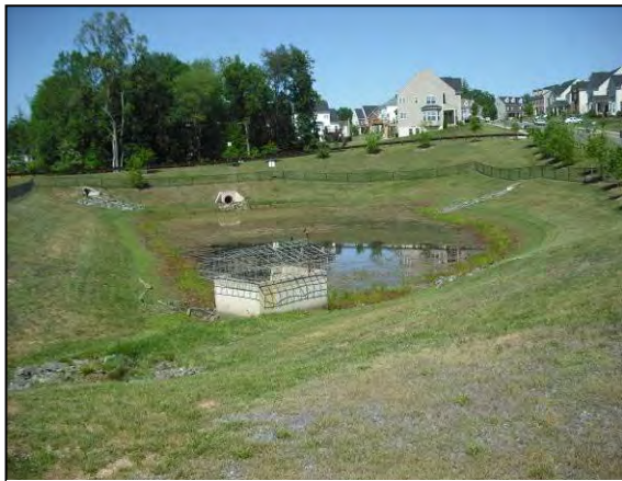
Figure 4-39: Wet pond in lacking forebay, microtopography, and vegetation, FAC-669.
