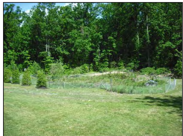
Figure 4-37: Vegetated basin, lacking internal structure and microtopography, FAC-5515.
