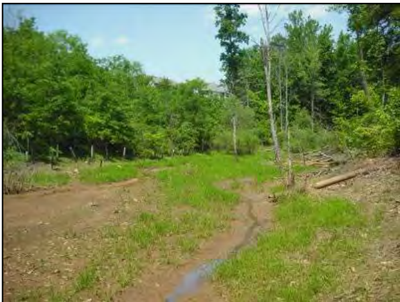
Figure 4-18: Sedimentation of inline basin, east of Oyster Bay Court, Reach 665-B.
