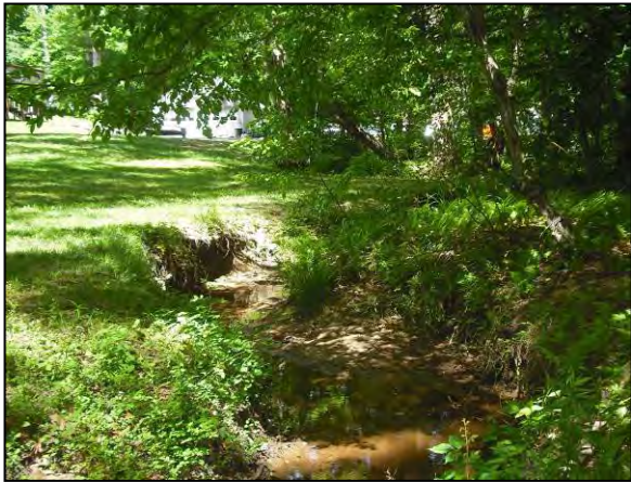
Figure 4-12: Removal of riparian forest and mowing to the top of bank, Reach 645-C.
