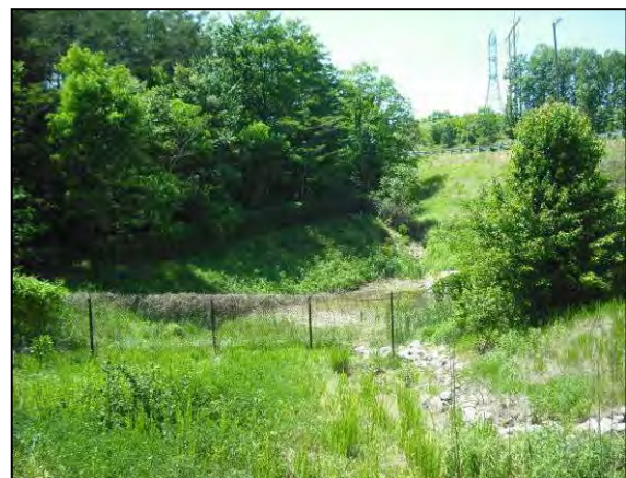
Figure 4-43: Steep gradient, riprap swales leading to the existing wet pond, FAC-5462.
