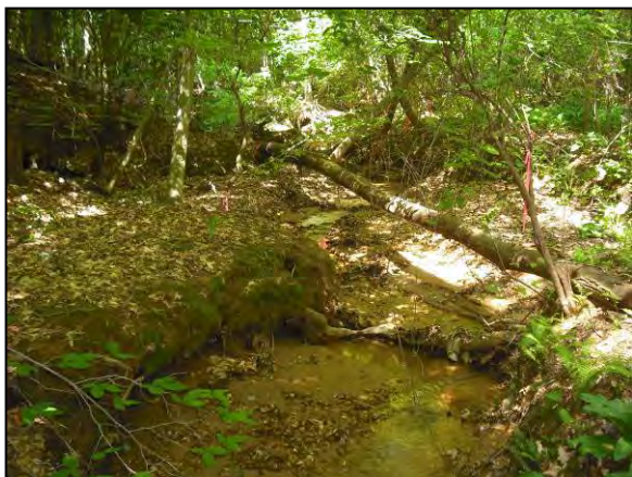
Figure 4-24: Deposition and channel widening, upstream from Myrtlewood Drive, Reach 665-H.
