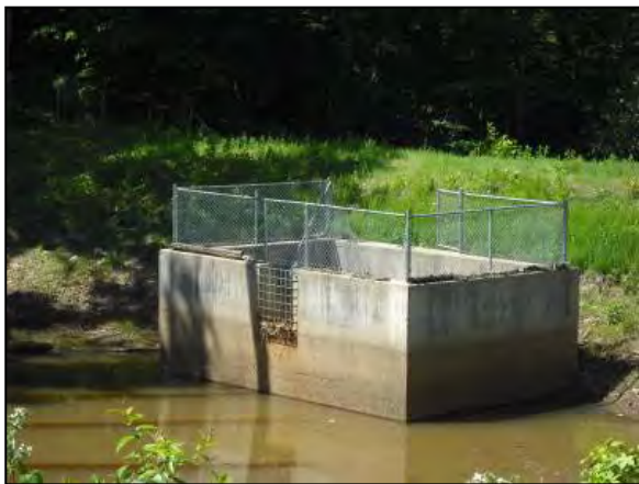
Figure 3-10: Existing Concrete Outlet Structure.
