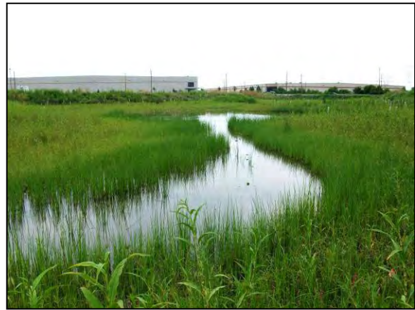
Figure 5-8: Example of pond microtopography, designed to lengthen the flow path.
