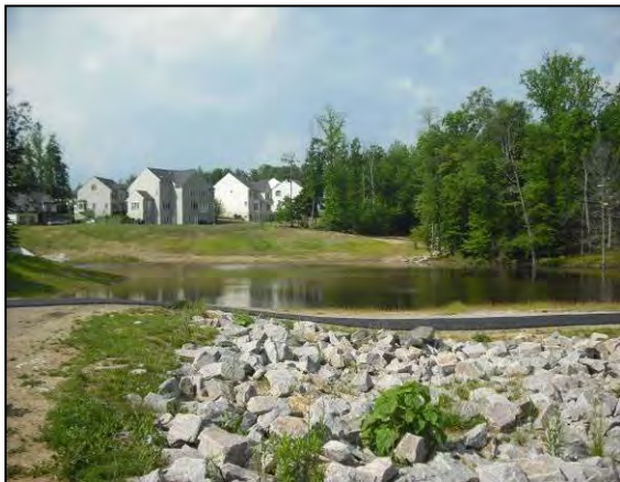
Figure 4-46: Pond with adequate storage capacity, lacking native vegetation, FAC-9025.
