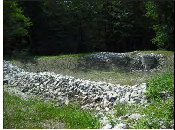
Figure 4-35: Dry basin lacking internal structure, microtopography and vegetation, FAC-5379
