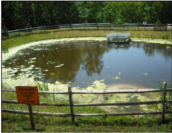
Figure 4-45: Existing wet pond, lacking forebay and native vegetation, FAC-Unknown.
