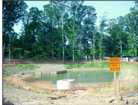
Figure 4-41: Newly constructed pond, lacking forebay and vegetation, FAC-5000.
