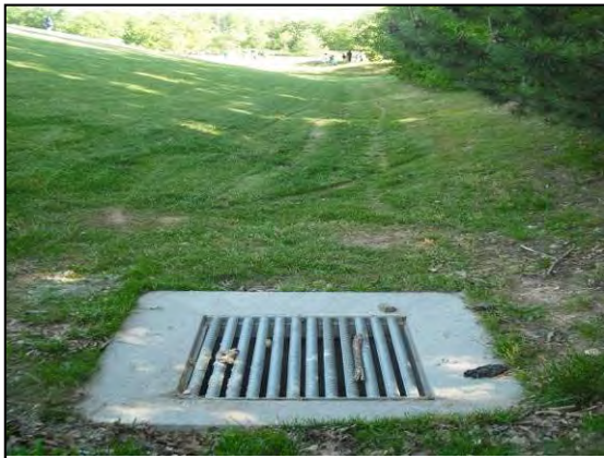
Figure 4-33: A grated inlet structure at the downstream end of the shallow swale,
