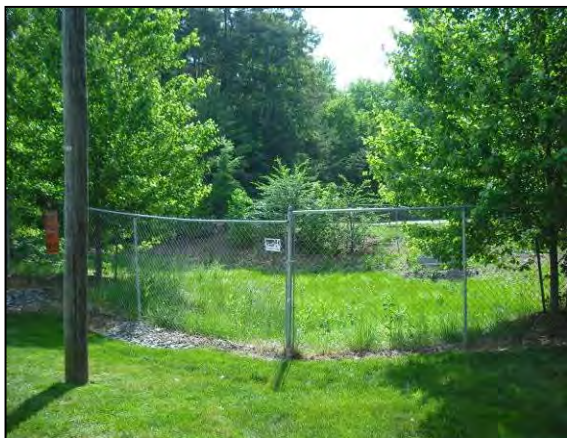
Figure 4-40: Well-vegetated extended detention basin, with short flow path, FAC-5397.
