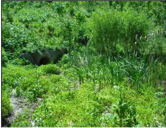
Figure 4-44: Extended detention basin with dense vegetative growth, FAC-505.
