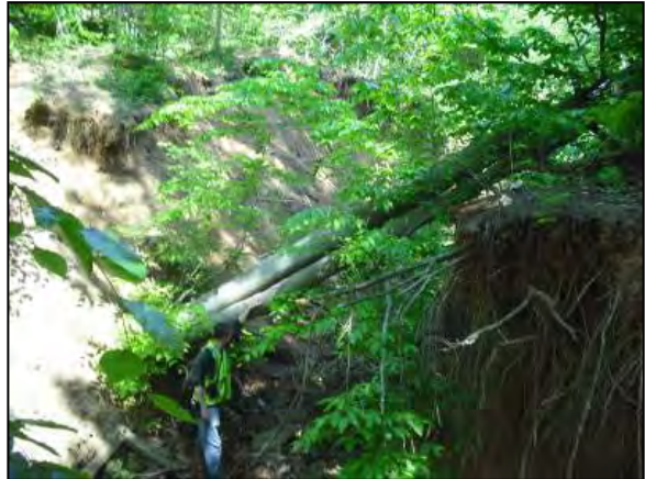
Figure 4-25: Severe channel incision and imminent loss of property, Reach 665-I.
