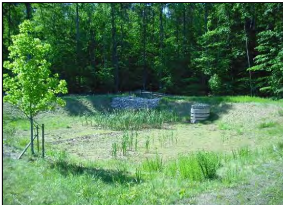
Figure 4-34: Dry basin lacking internal structure, microtopography and vegetation.
