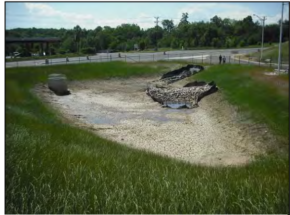
Figure 4-36: Newly constructed pond, with no permanent pool, and short flow path, FAC-5463
