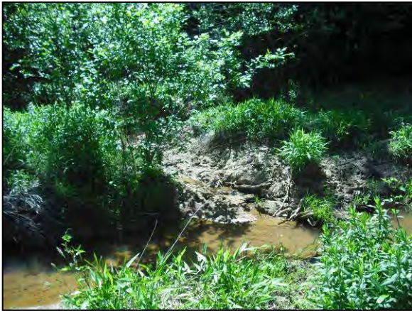
Figure 4-17: Channel incision and erosion near Crystal Downs Terrace, Reach 665-A.
