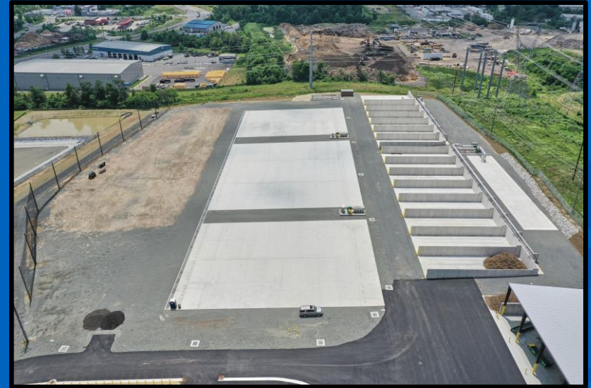
Balls Ford Road Compost Facility 13000 Balls Ford Rd., Manassas
