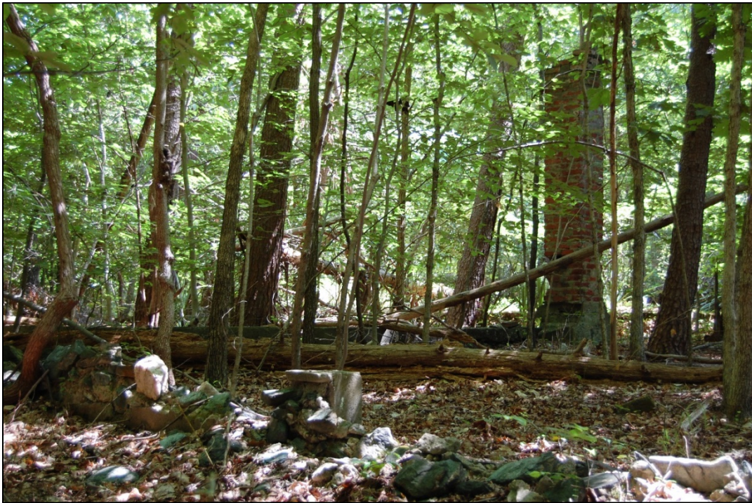
Foundation and chimney of Cabin Branch School, facing east toward Mine Road.
