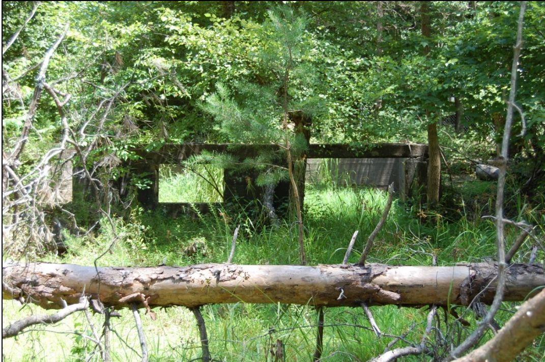
Cabin Branch Pyrite mine commissary building as seen from the pyrite mine trail in Prince William Forest Park.
