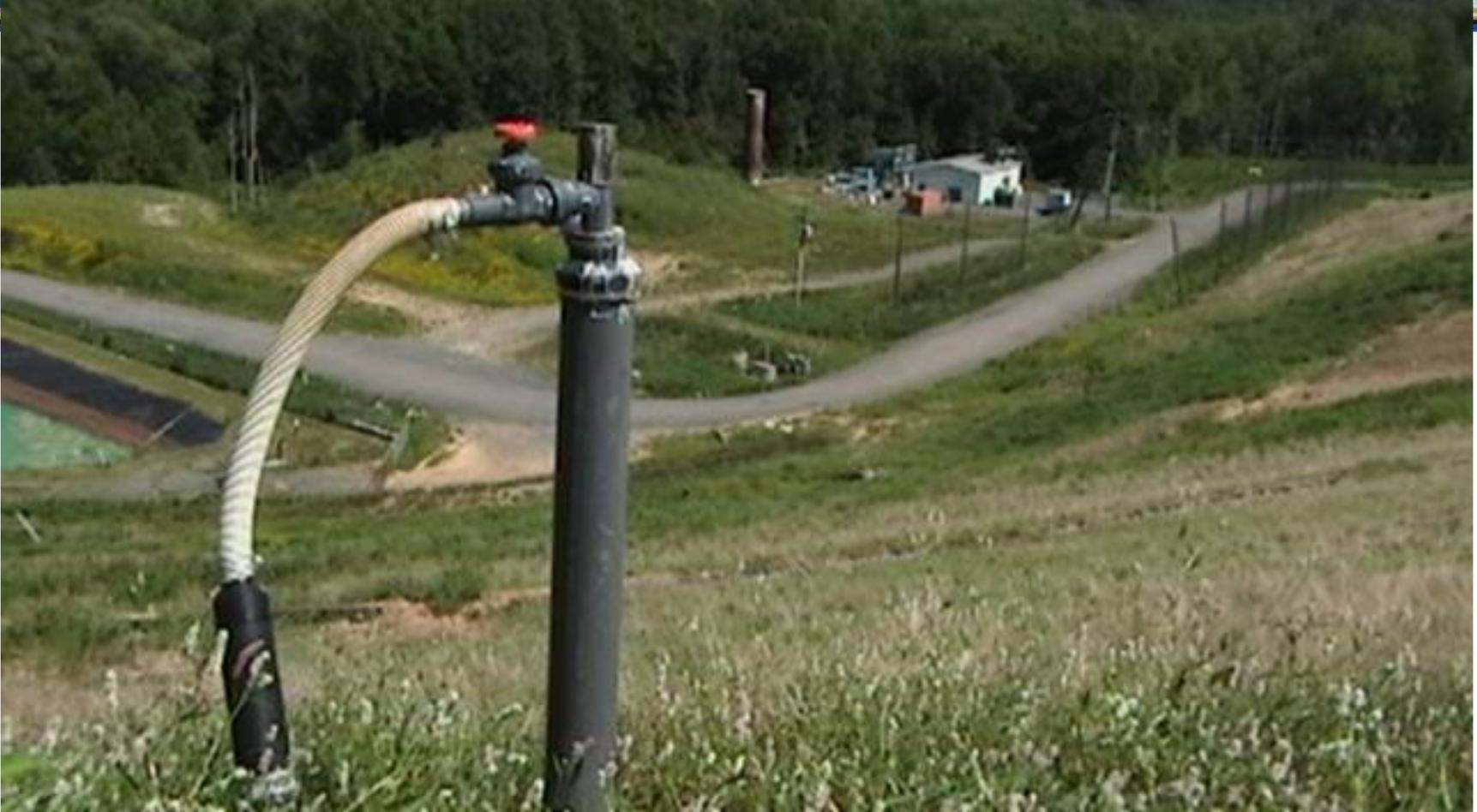
**The landfill has over 100 extraction wells for collection of landfill gas.**
