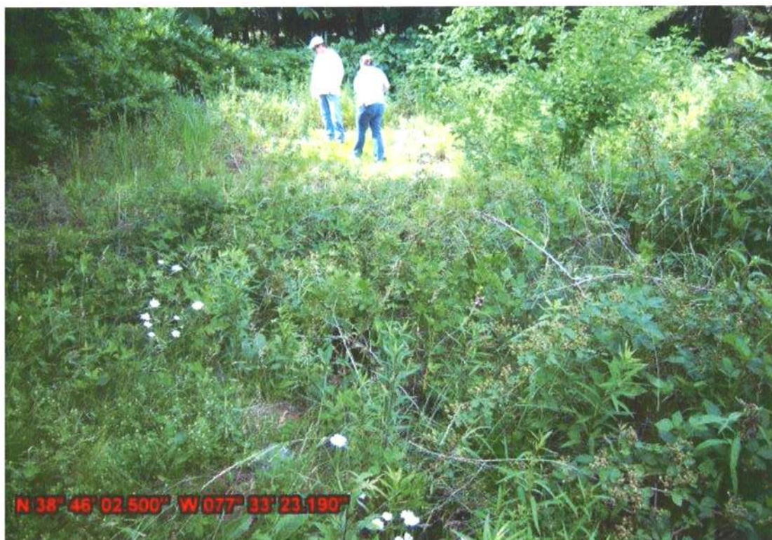
Photo 2: Basin not maintained and possibly filled
