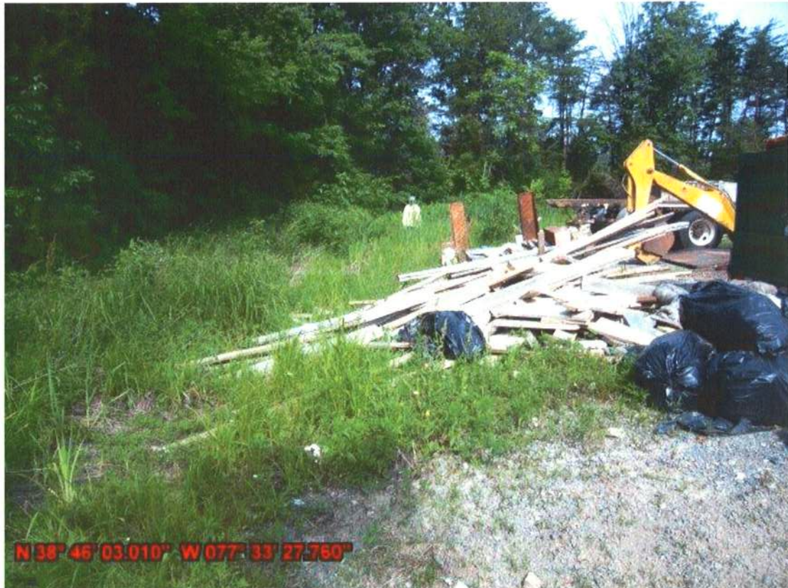
Photo 1: BMP facility appears to be partially filled by gravel parking and storage
