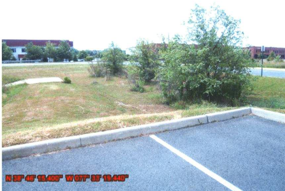
Photo 1: Bioretention forebay with under drains which discharge to dry basin
