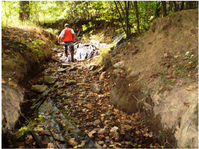
Outfall Channel from High School Stormwater Pond
