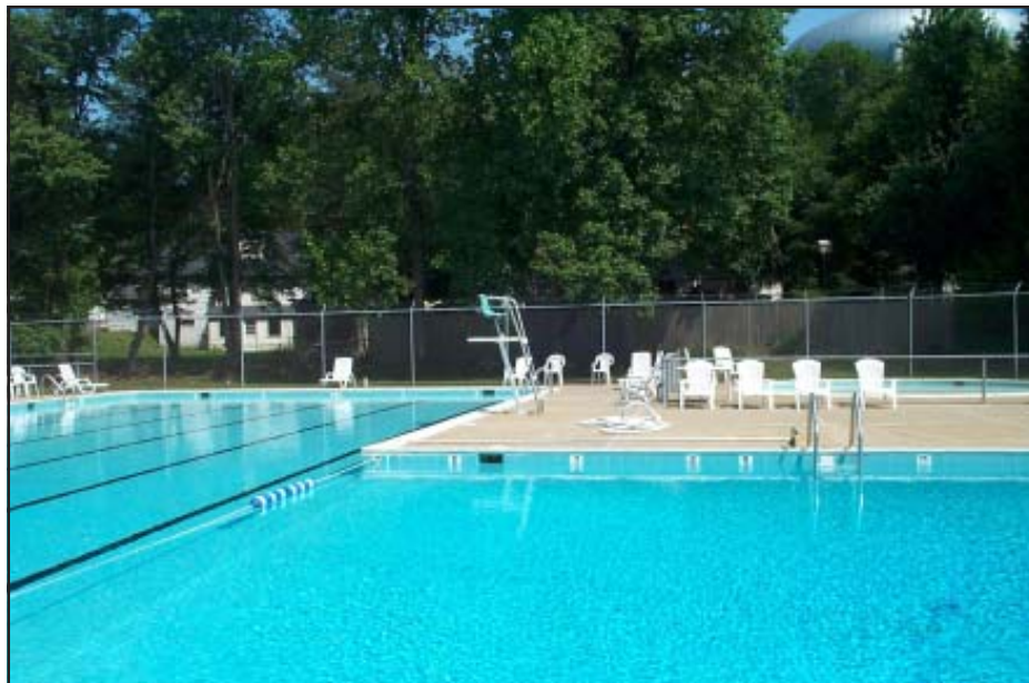
Hammill Mill Pool
